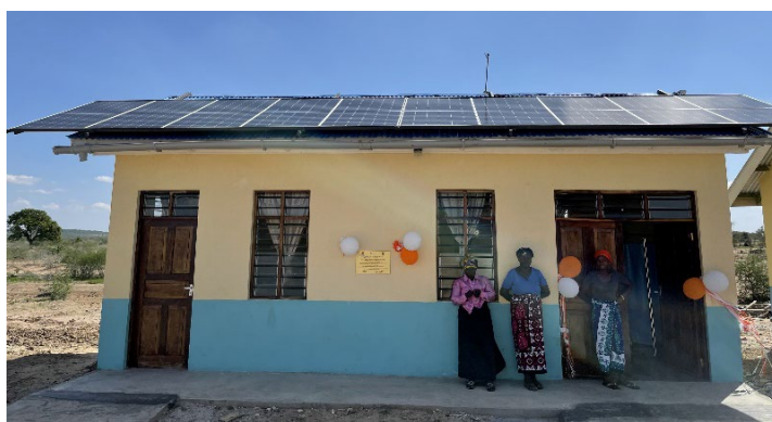
Maternity ward with solar panels installed
