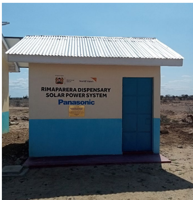
Solar power generation system
