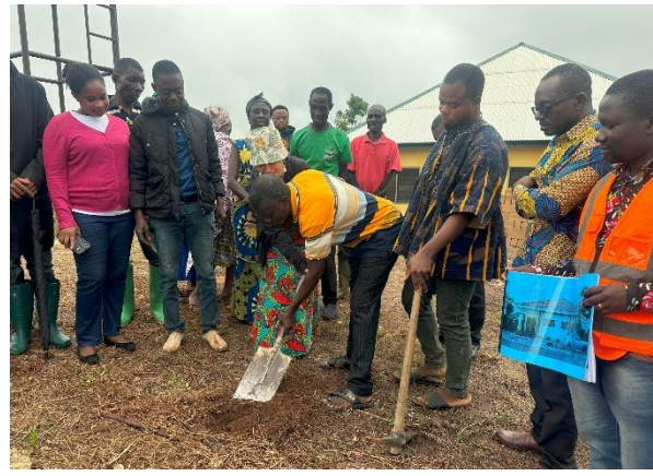
1-4 Construction of nurses quarter (Sutapong) (Photo: Ground-breaking ceremony, July 2025.)
