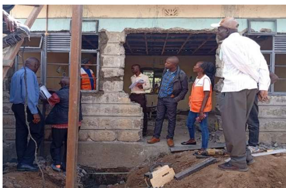
With engineers from Gil-Gil Sub-county Joint monitoring of maintenance work
