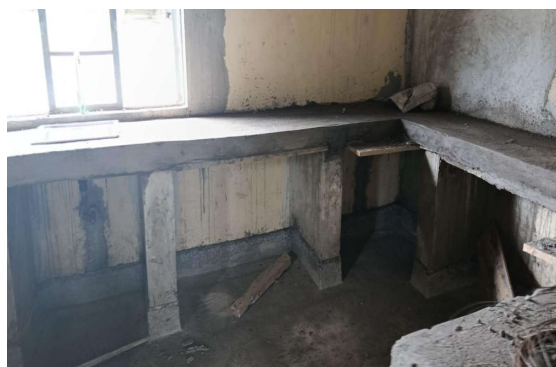
Newly installed Laboratory workbench
