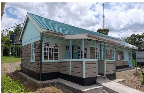
Maternal and Child Health Building and Laboratory near completion
