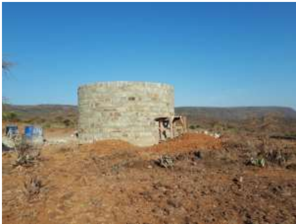
A water tank (under construction)
